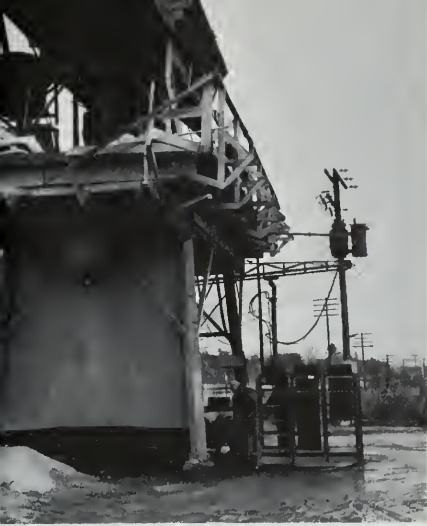
A concrete-block plant on Santee's lines is typical of small rural industries that are springing up in the electrified countryside.
